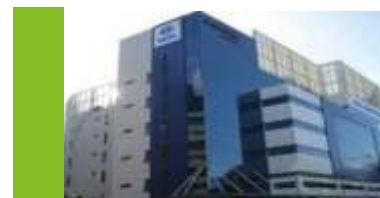
Tata Communications Exchange
