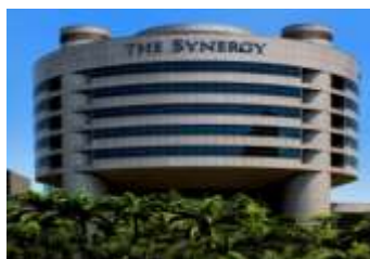
Business Park Buildings
